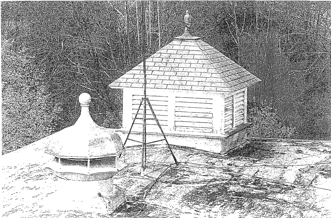
ROOF EXHAUST HOUSINGS - AT WEST END OF ROOF
