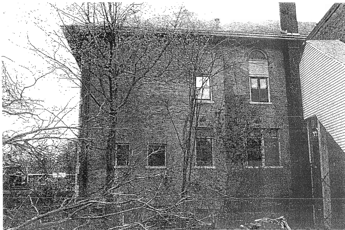
WARREN TOWN HALL REAR (WEST) SIDE
