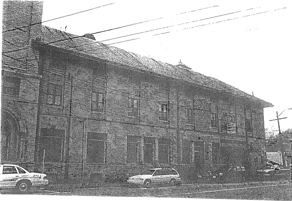
SLOPED (MAIN STREET) SIDE OF ROOF WITH SLATE SHINGLES
