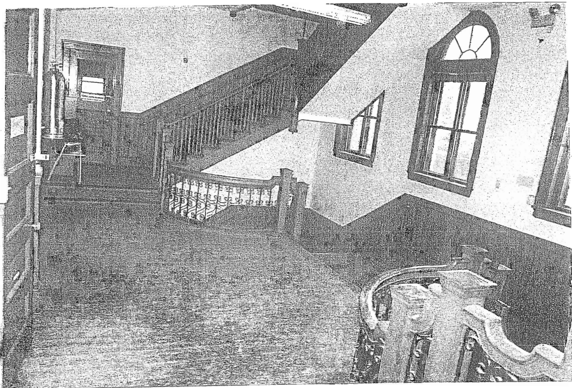
AUDITORIUM LEVEL ABOVE MAIN ENTRANCE LOBBY - STAIR BEYOND LEADS TO BALCONY
