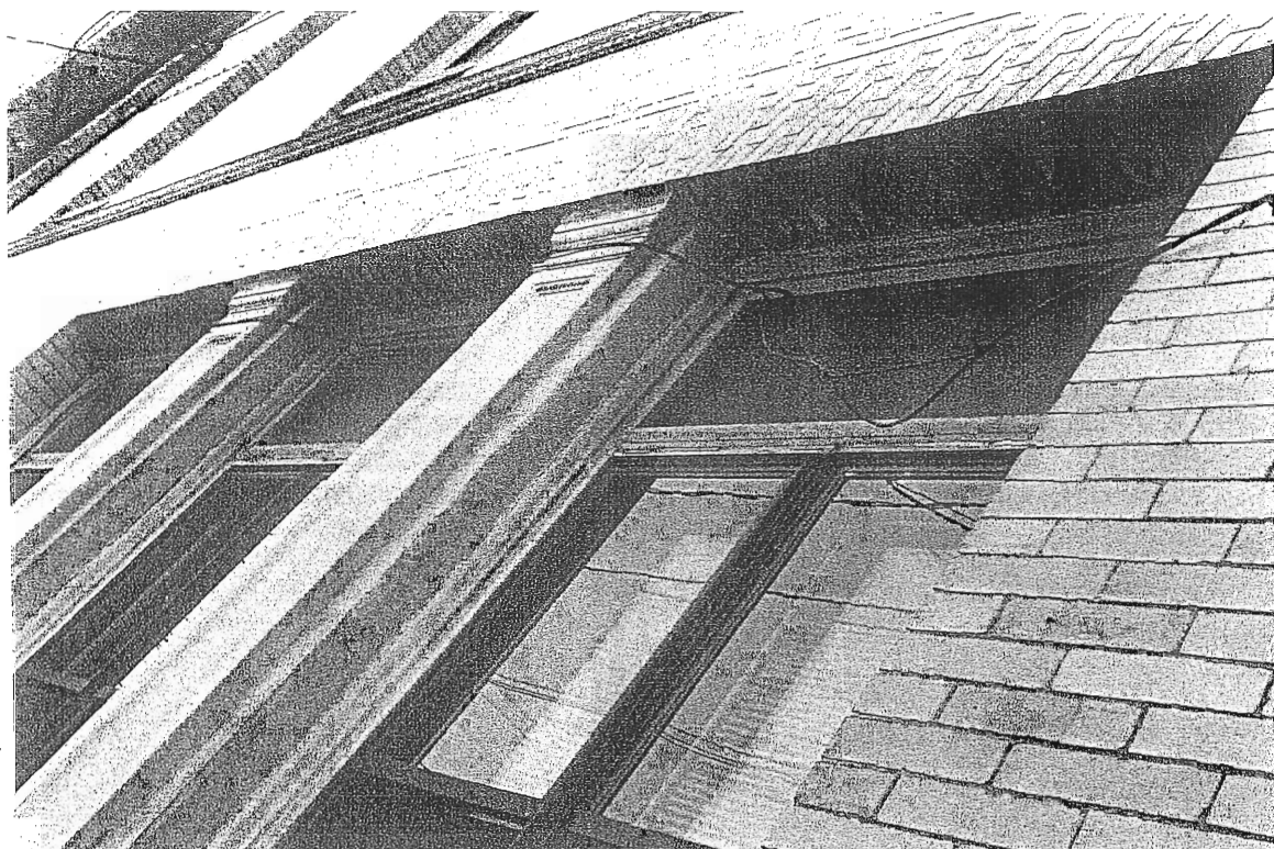
TYPICAL PALLADIAN WINDOWS MAIN ST. SIDE - NOTE RUSTING COMING TO SURFACE AT PILASTER SIDES
