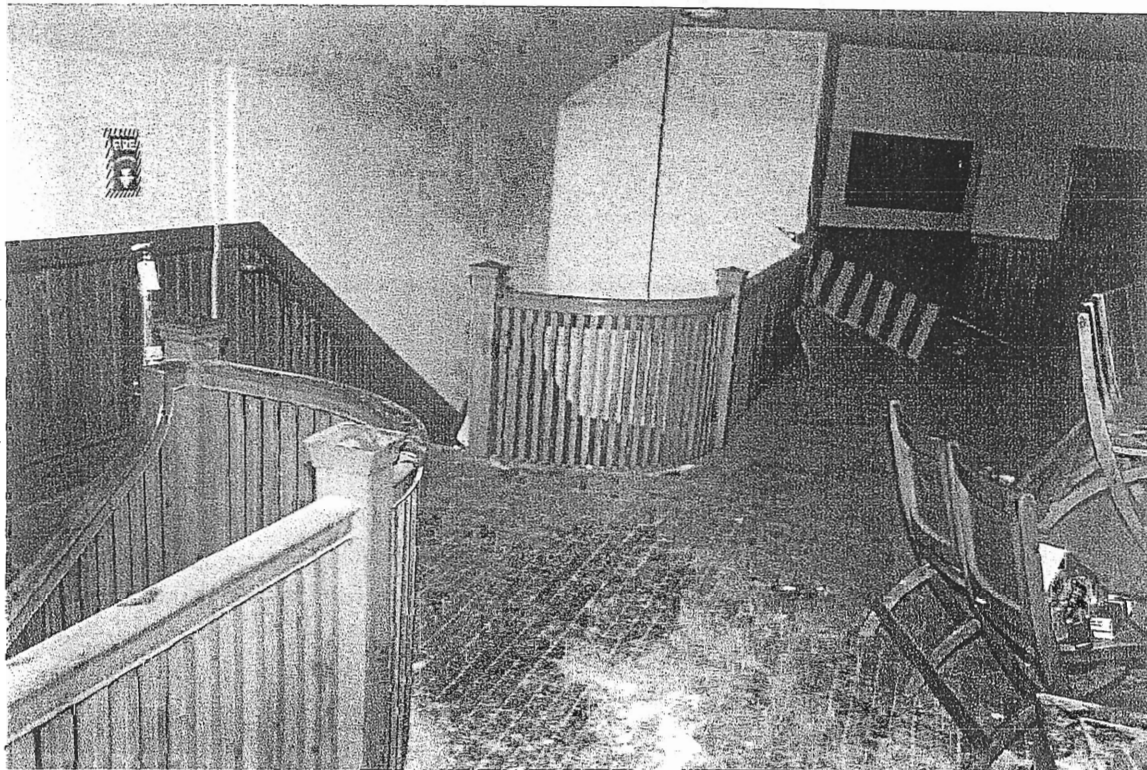
BALCONY LEVEL OPEN STAIRWAY AT LEFT AND CENTER
